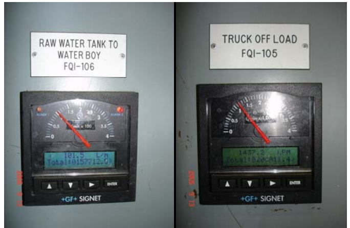
Figure 4. Water Supply. WSF Deep Lake raw water meter and entrance signage.
