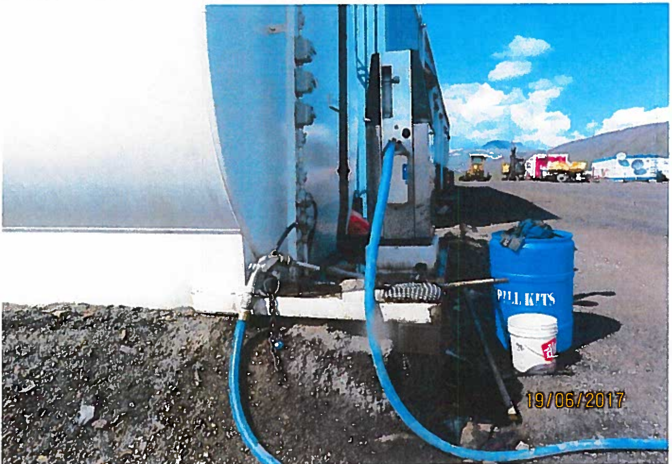
Figure 6 Fuel storage and transfer area, with no secondary containment
