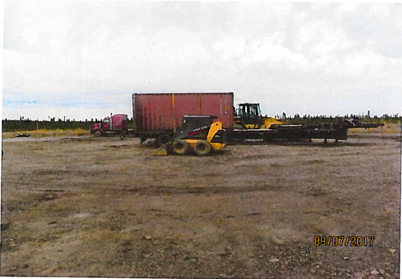
Equipment on site
