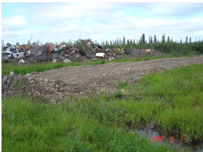
Figure 1 Berm around the Bulky Metal Waste Disposal Area.
