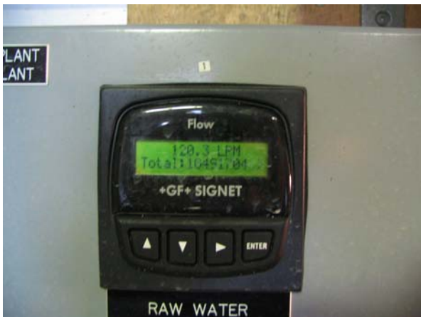
Figure 3. Water Supply. Water intake meter.
