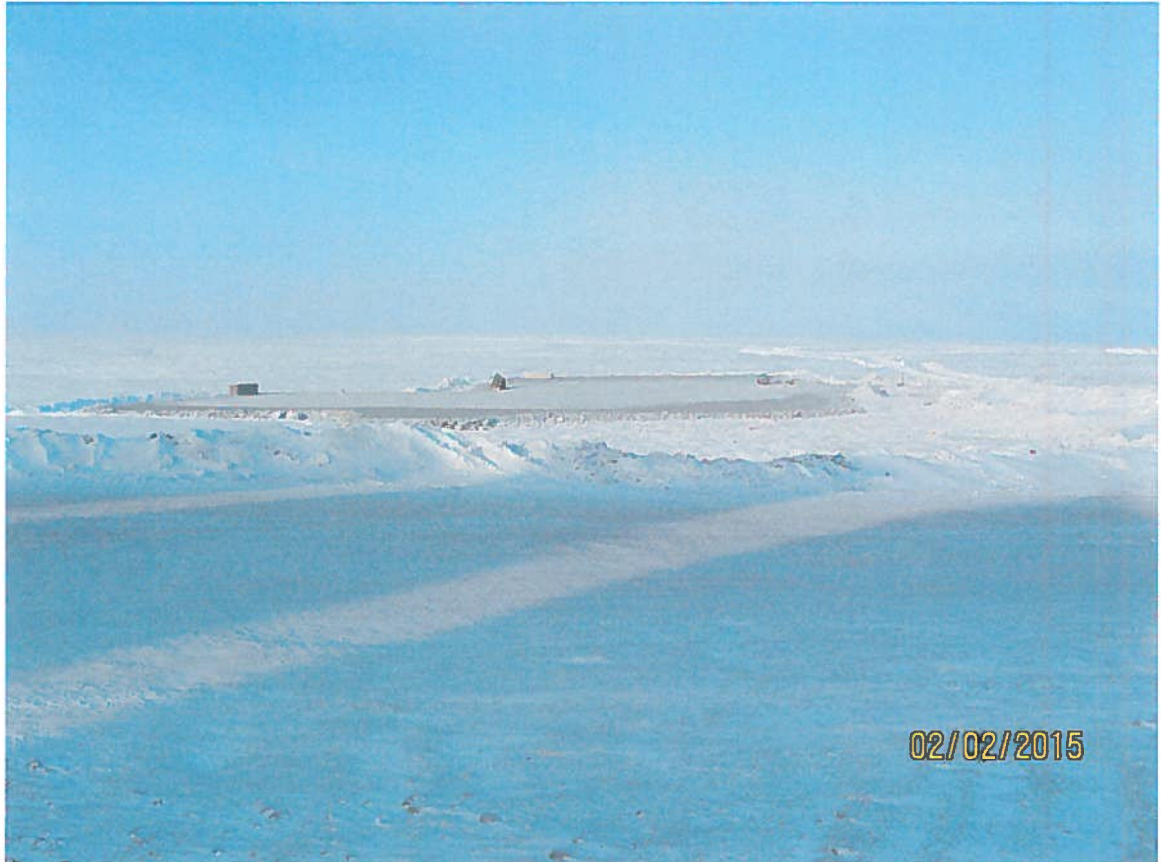
Figure 5. Construction of the “North Laydown Area”.
