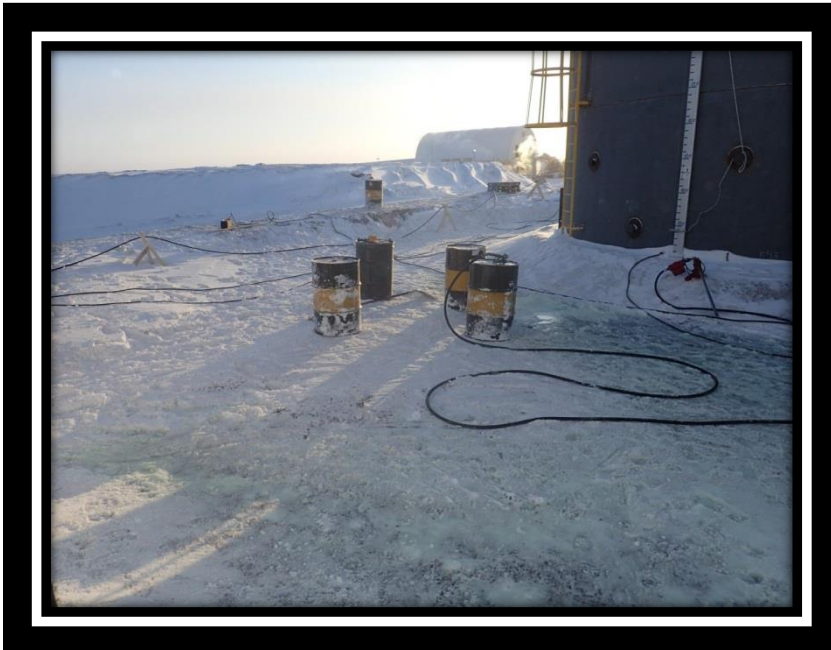
Photo 2 – Clean-up Operations In Process Using Pumps and Drums for Containment
