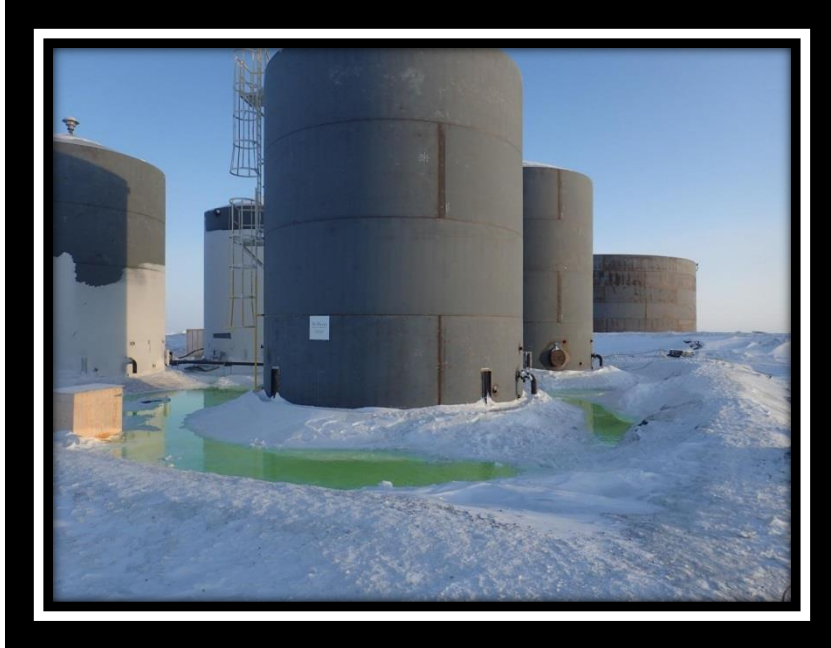
Photo 1 – Free Product Within Lined Containment Day After Spill
