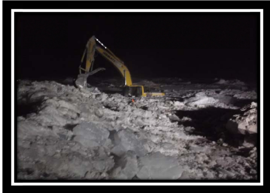
Photo 1 – PC-390 Excavator Positioning After Breach Through Ice
