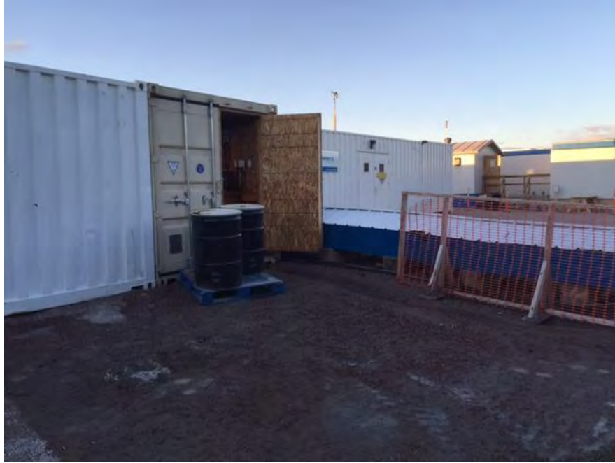
a. Location of spill outside of Emergency Overflow Lift Station (building with open door)
