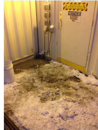
Oct. 16, 2014 – Photo of spill outside STP
