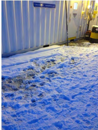
Oct. 16, 2014 – Photo of spill outside STP
