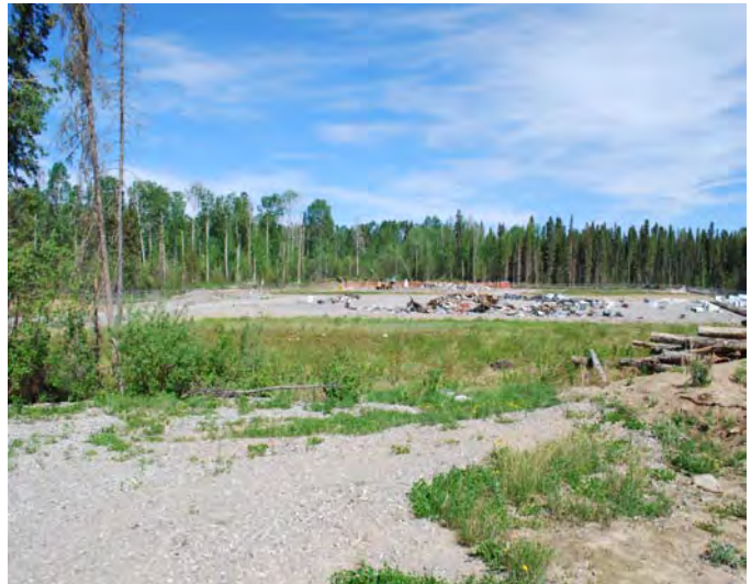
Figure 4 June 5th - new landfill site
