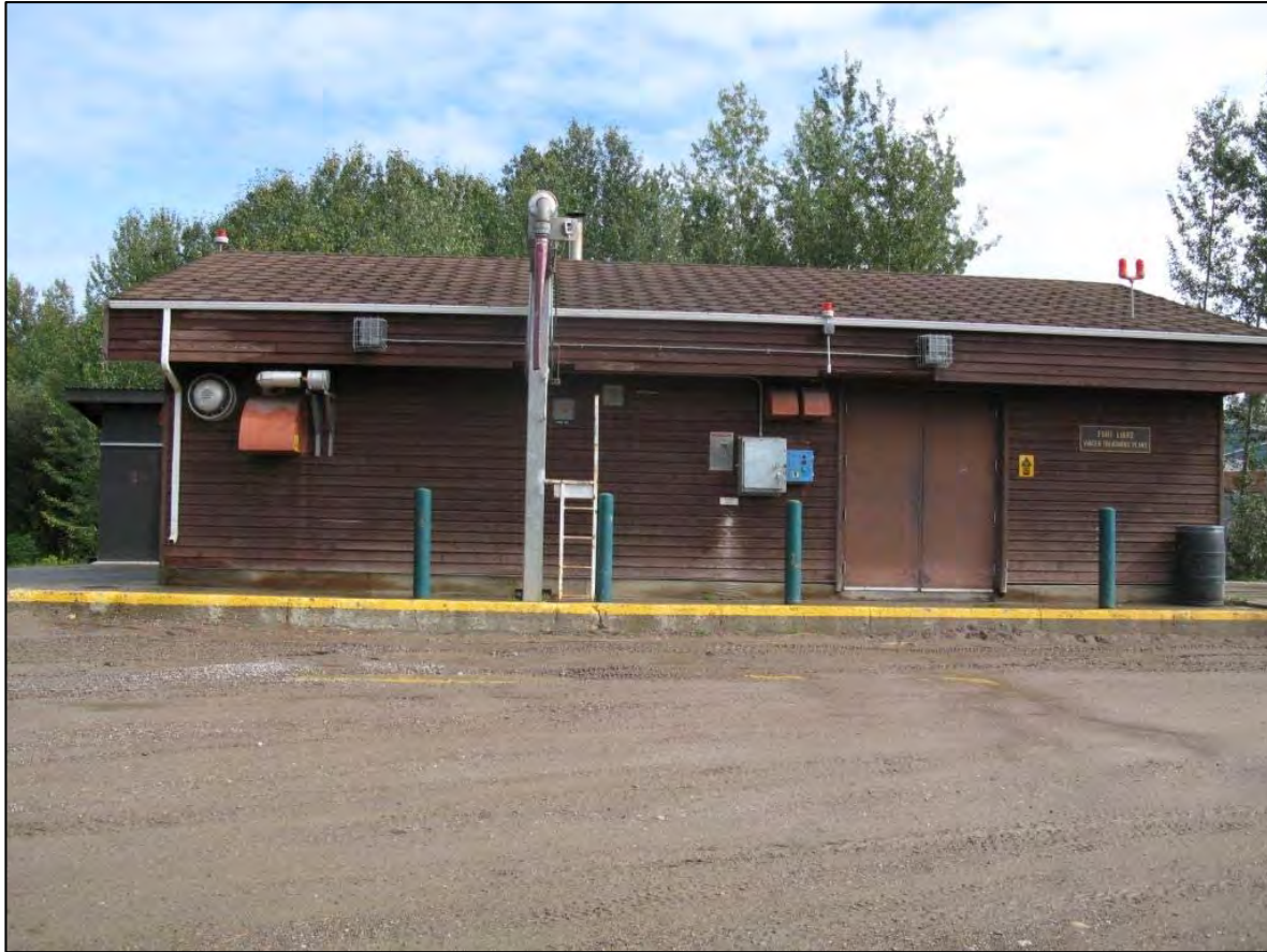
Figure 1 Hamlet of Fort Liard Water Treatment Plant.
