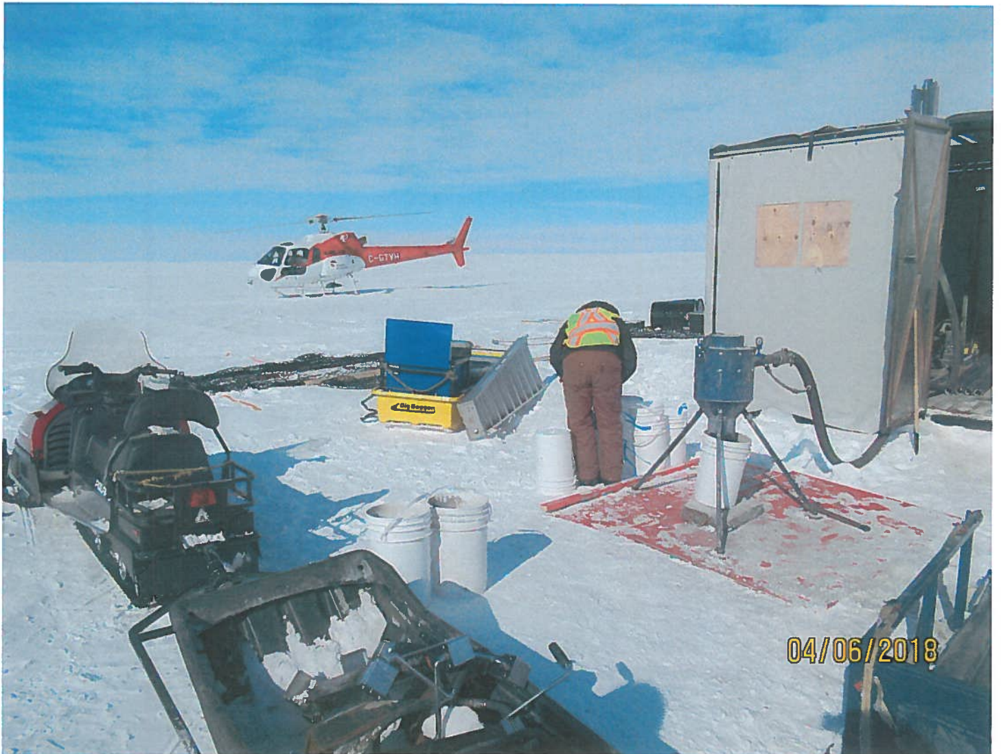
Photo #3 - MV2012C0009 - Dominion Diamond Mines ULC A centerfuge is being used to segregate and containerize drill cuttings into 5 gallon pails.
