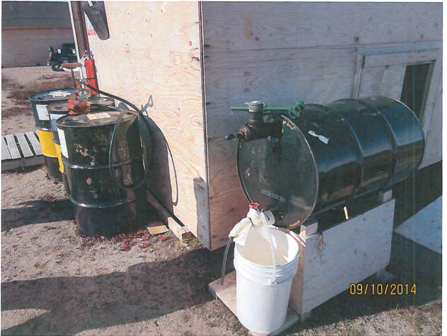
Photo #3 - MV2012C0009 - DDEC Mineral Exploration - Lac de Gras Area, NT Well maintained, covered grey water line and sump from camp kitchen.
