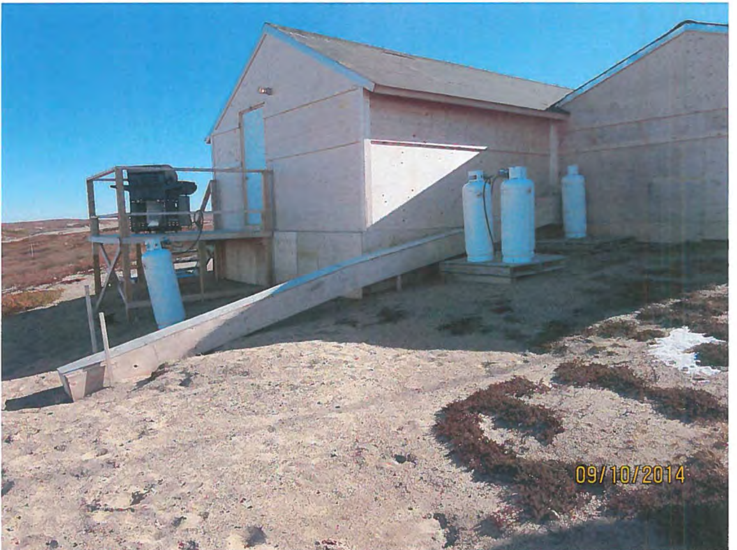
Photo #4 - MV2012C0009 - DDEC Mineral Exploration - Lac de Gras Area, NT Well maintained, covered grey water line and sump from camp kitchen.
