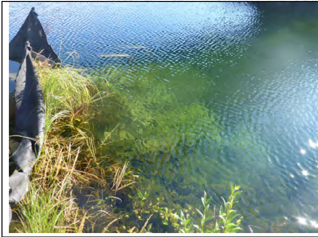
Photo 5: View directly underneath the west side of the bridge. Note the greenish/brown area under water where the sediment settled.
