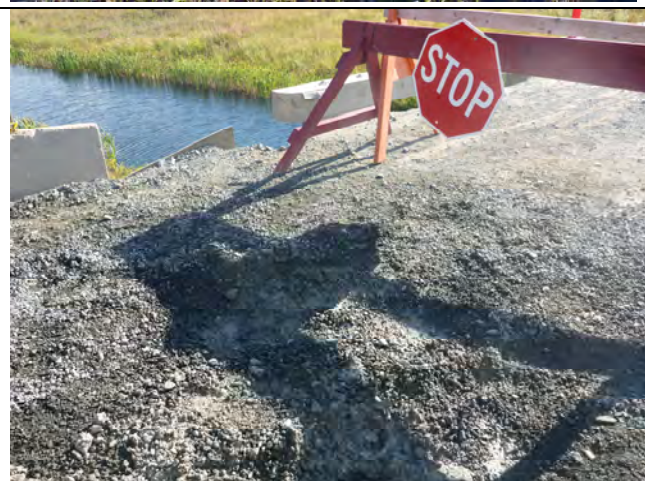
Photo 4: Close up of the drill location.
