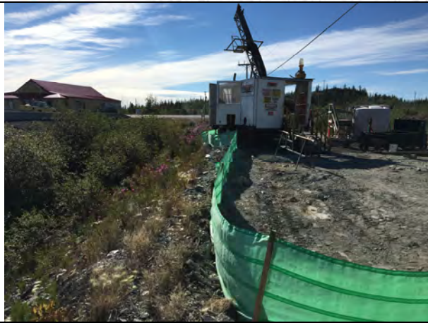
Photo 1: A1 Drill Site with Silt Screen
