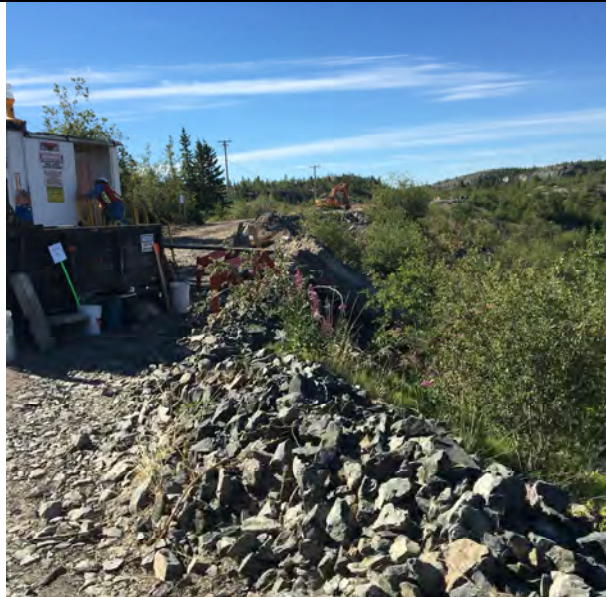
Photo 4: Cuttings being pumped into adjacent Pit from C1
