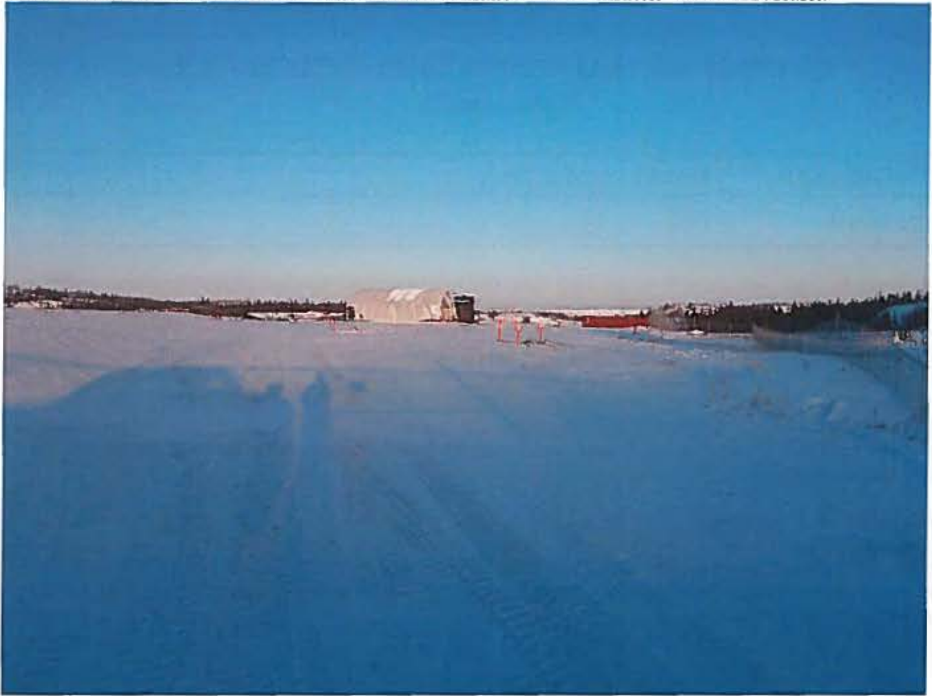
Photo 1 – Overview of the Roaster site after the demobilization of the contractor for the 2014 season
