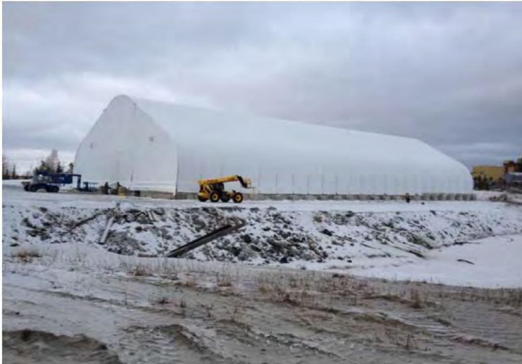
Figure 1 – Temporary Stockpile Building (CARD, 2017)
