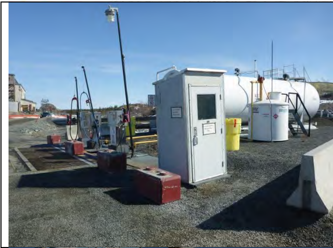
Photo 6: Fuel Transfer area
