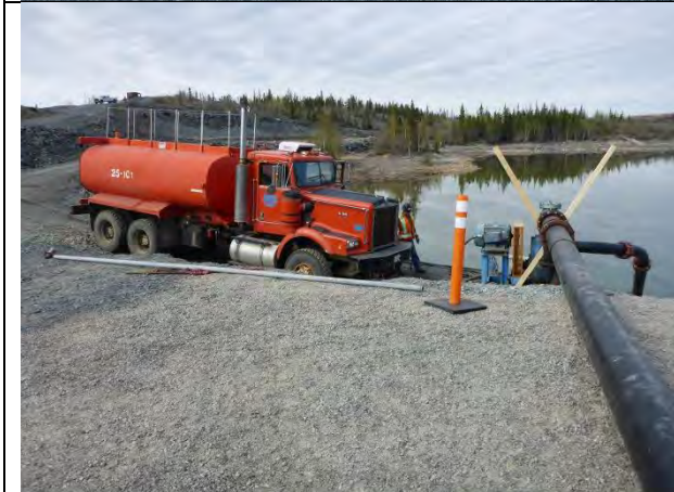
Photo 3: Pump truck pumping water for dust suppression
