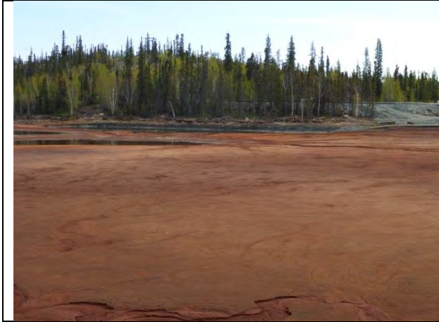
Photo 4: Overview of Polishing Pond
