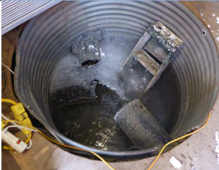
Photo #6: SNP station 4-12 discharging at the time of the inspection.
