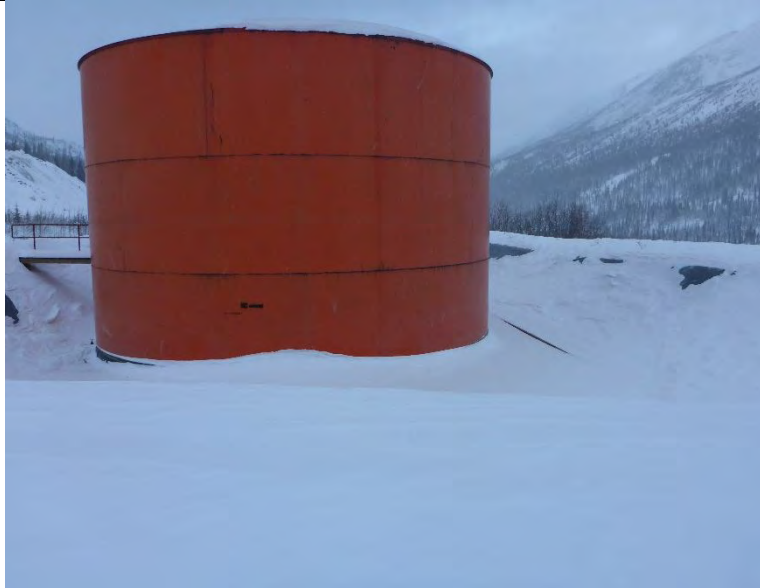
Photo #5: Large orange fuel tank located uphill from the mill.
