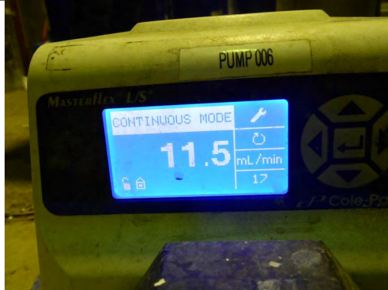
Photo #2: Chlorine injection rate at the water treatment plant.
