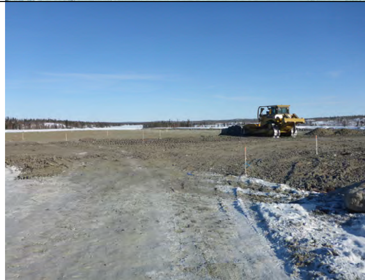
Photo #6: Overview of the tailings cap on Camlaren.
