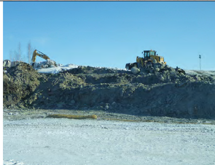
Photo #5: Overview of the excavation of waste rock at Camlaren.
