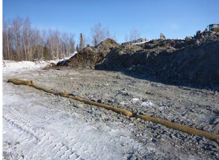
Photo #4: Overview of the excavation of waste rock at Camlaren.
