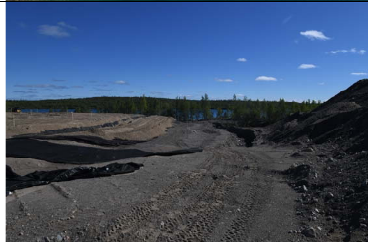
Photo #5: Overview of the excavation of waste rock at Camlaren.
