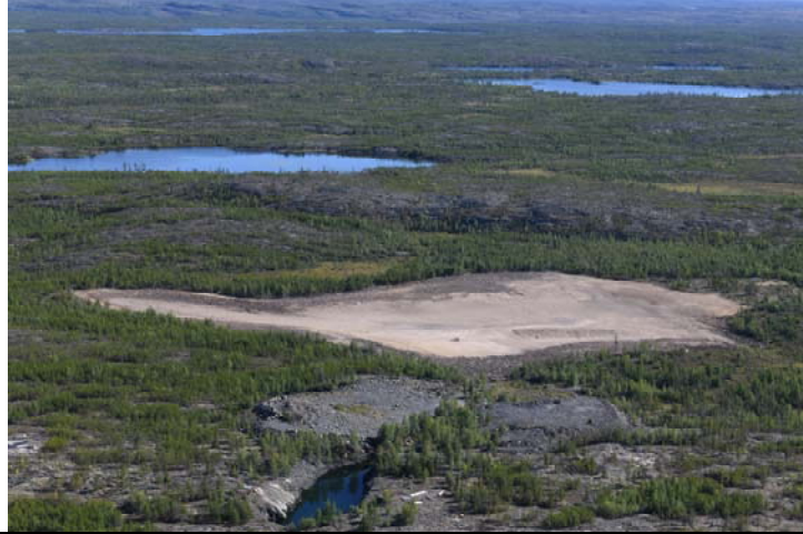
Photo #7: Overview of the remediated quarry at Westbay Mine site.
