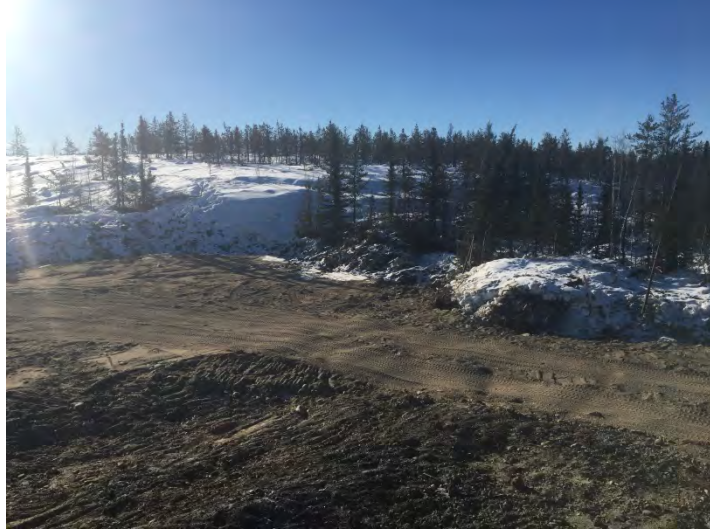
Photo #4: Overview of Treacy and excavation.
