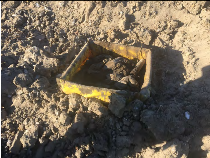
Photo #5: Spill pad at West Bay with contaminants sitting between two pieces of equipment with no drip tray.
