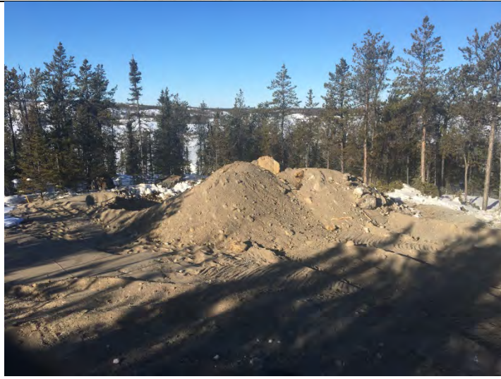
Photo #1: Stockpile of clay and rock at Kidney Pond.
