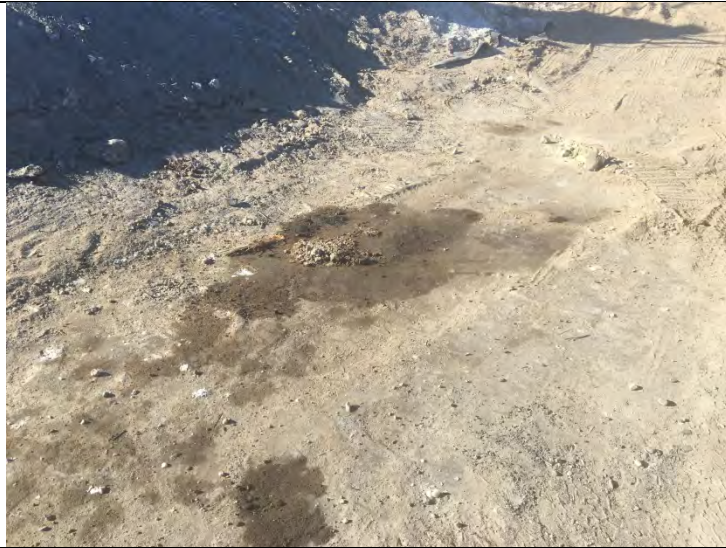
Photo #9: Fuel stains behind the fuel berm at Camlaren.
