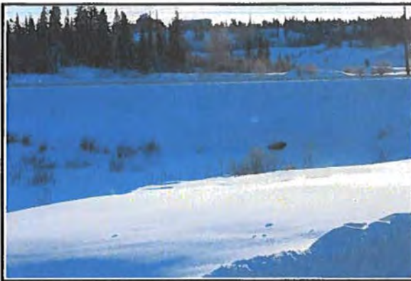
Location: Trapper Cr. Culvert #1
