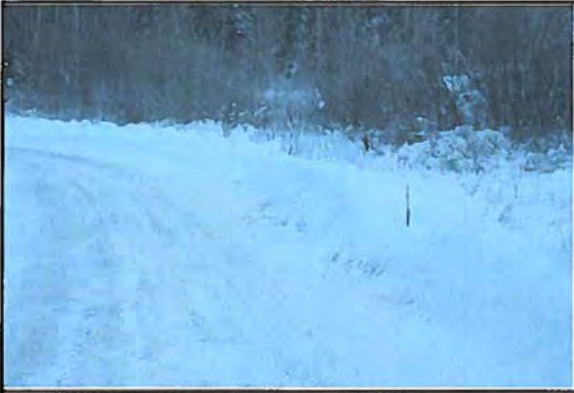
Location: Trapper Cr. Culvert #3
