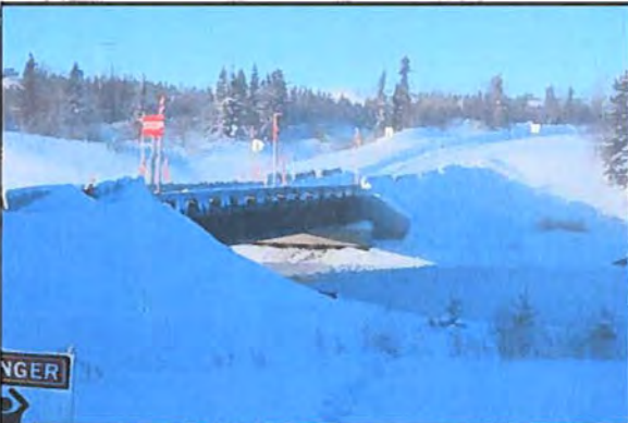
Location: REACH 4 - UBC Bridge
