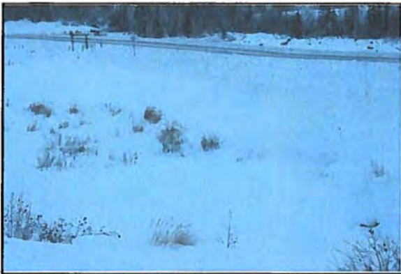
Location: Trapper Cr. Culvert #1
