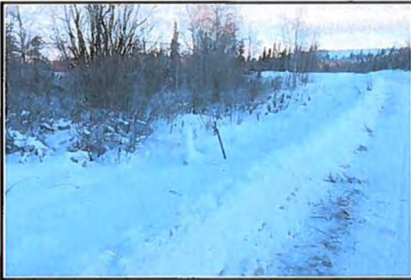
Location: Trapper Cr. Culvert #3
