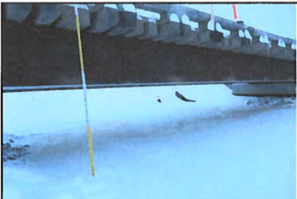
Location: REACH 4 - UBC Bridge
