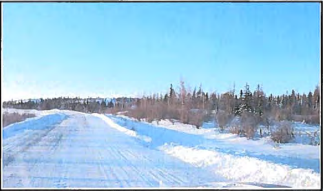
Location: Trapper Cr. Culvert #4
