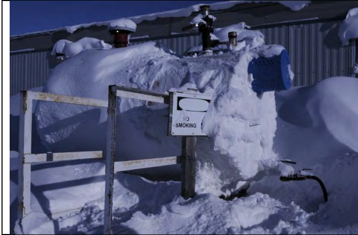
Photo #1: Photo of Fuel tank for camp with fuel stains on the side of the tank and on the bottom. This snow must be removed and placed in proper containment.
