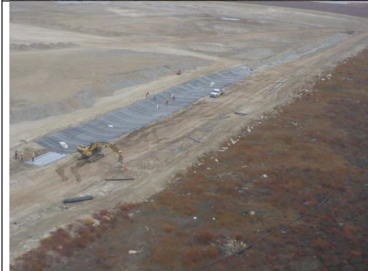
Photo #3: Tailings contaminated area diversion ditch construction.
