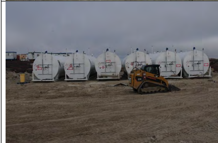
Photo #9: New tank farm berm with new empty tanks placed inside.
