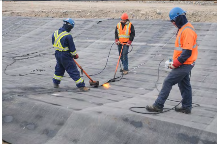
Photo #12: Seams of the liner being welded together.
