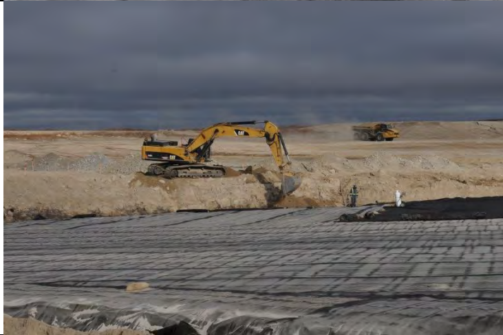
Photo #15: Dirt being placed on top of the tailings cap membrane.
