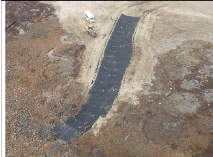
Photo #2: Mill Pond outflow construction.
