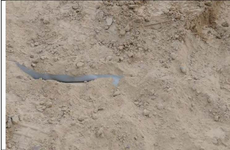
Photo #19: Liner on the berm edge.
