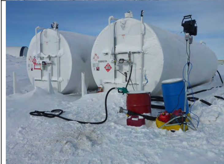
Photo #8: The two 100,000 liter tanks remaining onsite.
