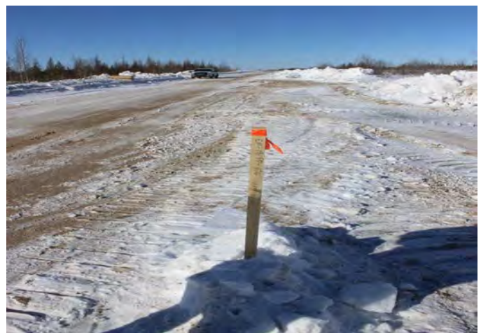
Figure 6 EM-18-PP-106. This is the next hole to be drilled on access road. Note that these holes are on the road surface and need to filled to prevent any public safety issues.
