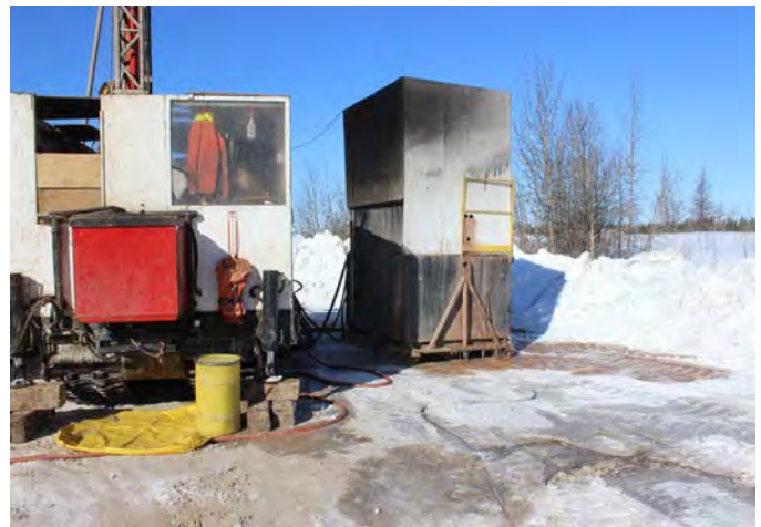
Figure 6 EM-18-PP-106. This is the next hole to be drilled on access road. Note that these holes are on the road surface and need to filled to prevent any public safety issues.
