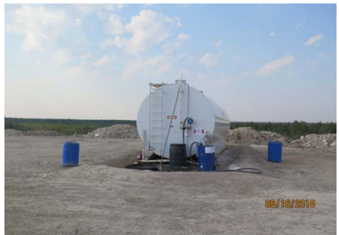
Figure 12 50,000L double-walled fuel tank.
