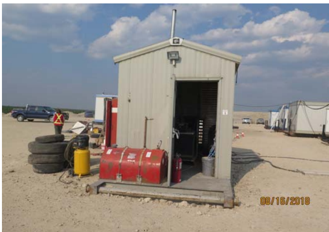
Figure 11 Generator shed with 400L single-walled fuel tank.
