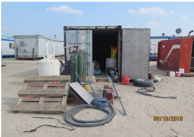
Figure 11 Generator shed with 400L single-walled fuel tank.
