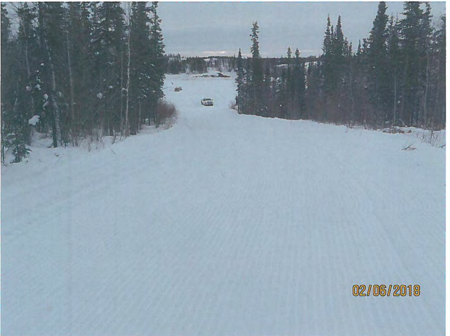
Photo #2 - MV2017X0005 - NTPC - Bluefish Winter Road Southern ramp onto the first portage is being iced by hand and a water truck will be mobilized on Feb 7, 18.
