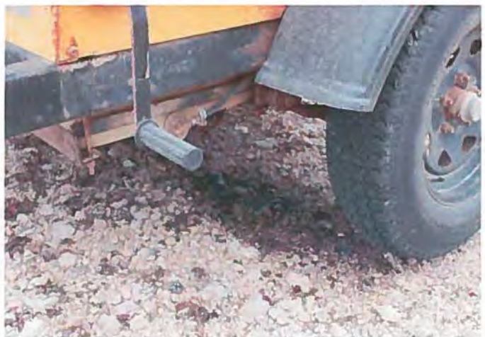
Figure 12 Leak under generator
