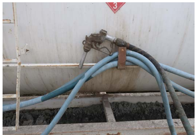
Figure 12 Km 241.5 - Refuelling nozzle requires containment.
