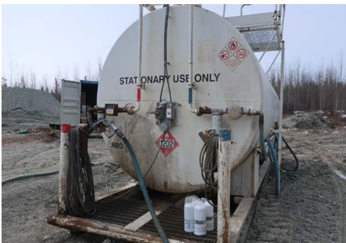
Figure 11 Km 241.5 - 34,000L Double walled fuel tank.
