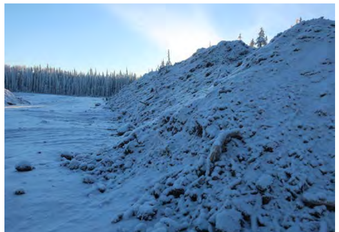
Figure 12 Km 204.9 - Windrowed overburden on the west side of the clearing.
