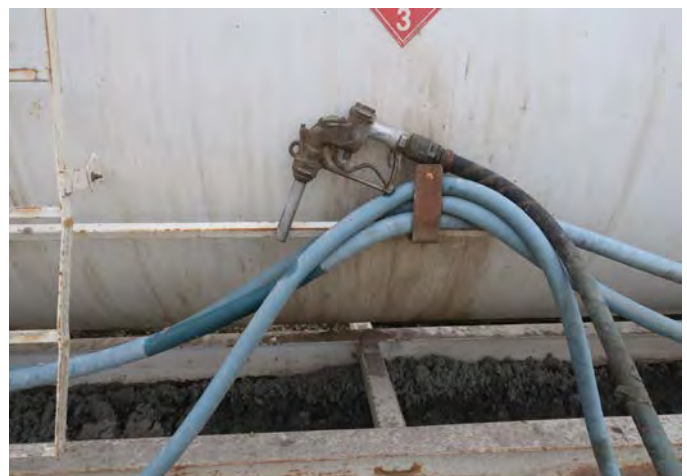
Figure 12 Km 241.5 - Refuelling nozzle requires containment.
