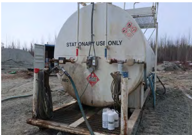
Figure 11 Km 241.5 - 34,000L Double walled fuel tank.
