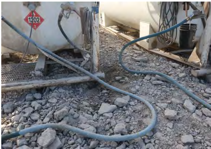
Figure 17 Small spill next to fuel tank.
