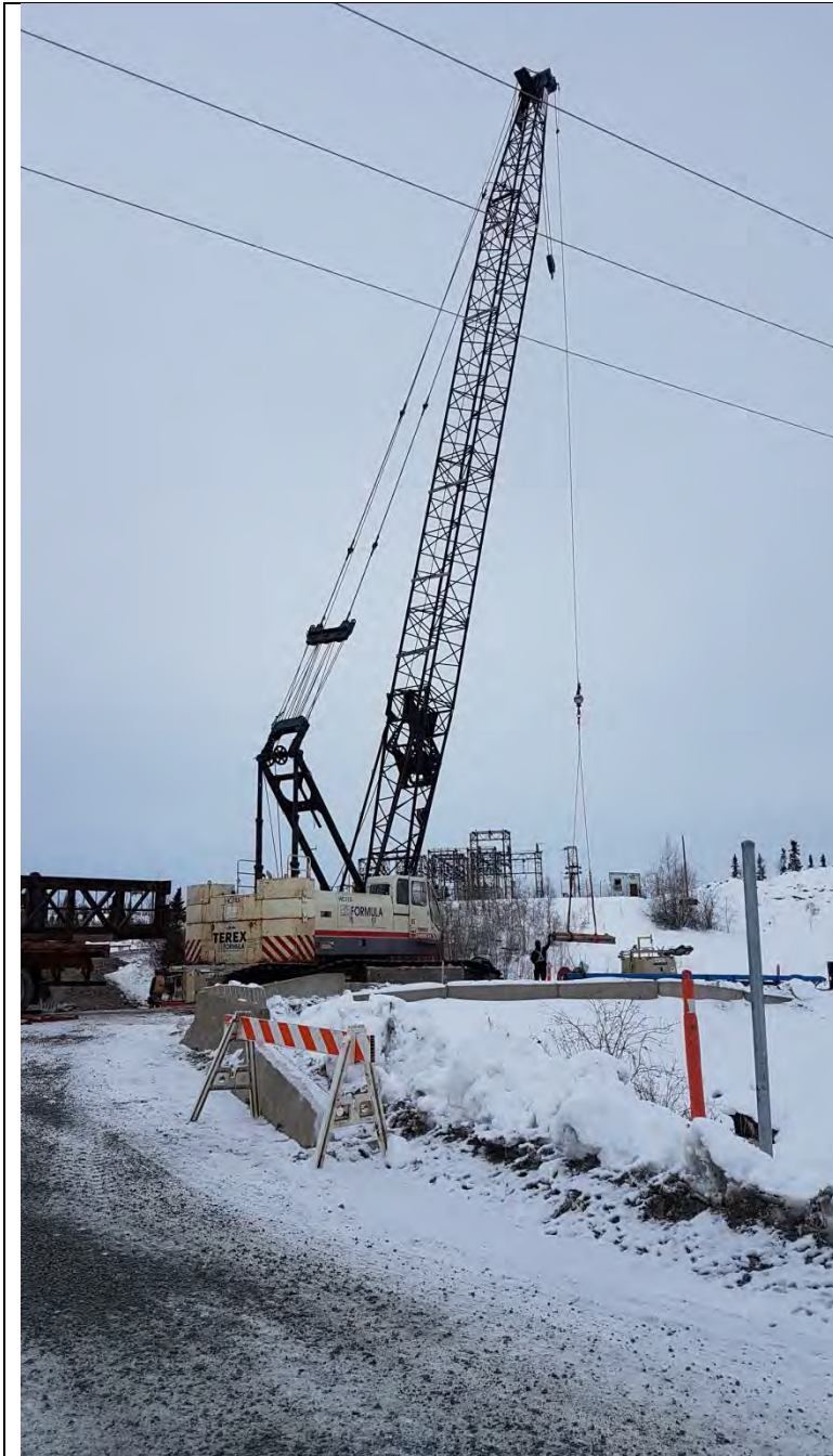
Photo #1: 110 Ton Crane used in the repair of the bridge
