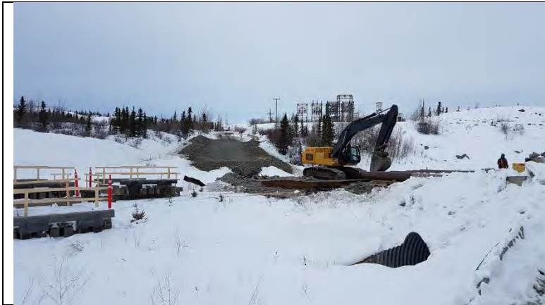
Photo #4: Overview of the bridge area that spans Baker Creek.
