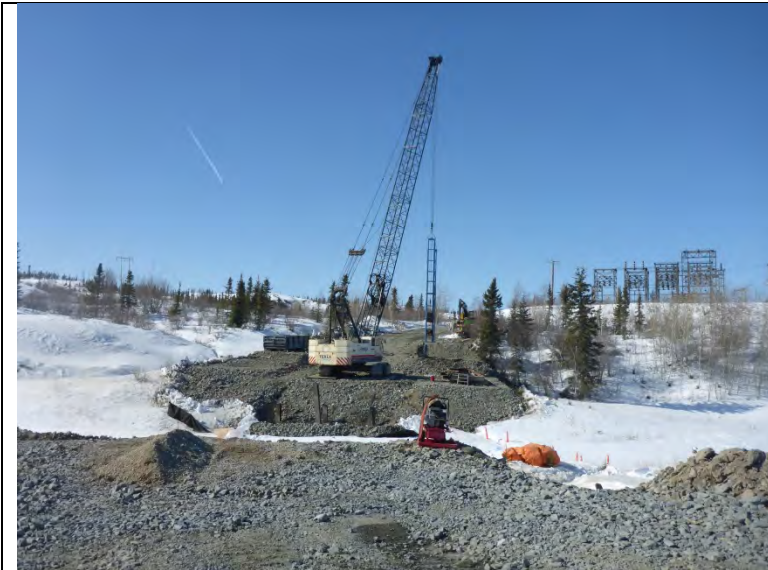
Photo #1: 110 Ton Crane moved to the west side of the bridge.
