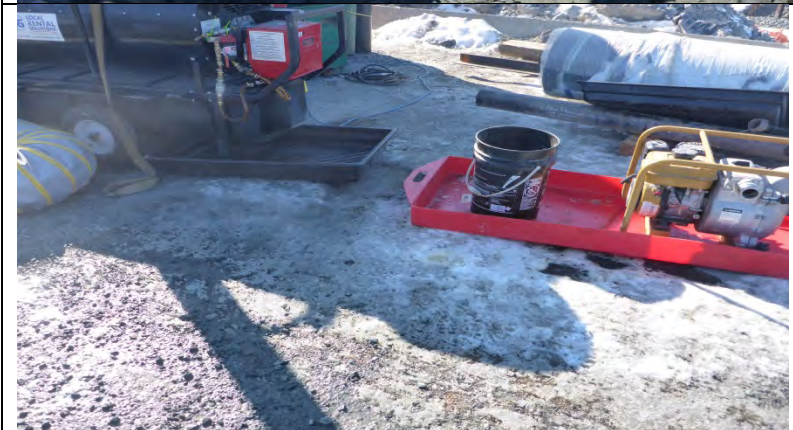
Photo #3: Secondary containment under machinery containing fuel.
