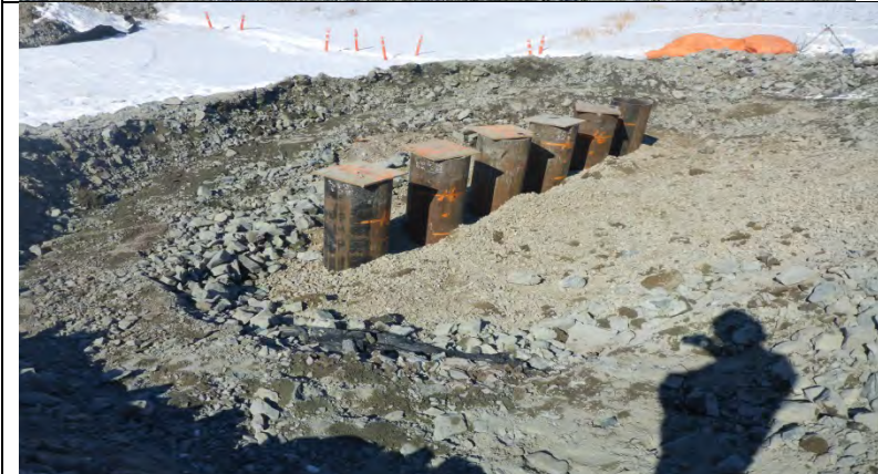
Photo #2: 6 New 20" piles on the east side of Baker Creek.
