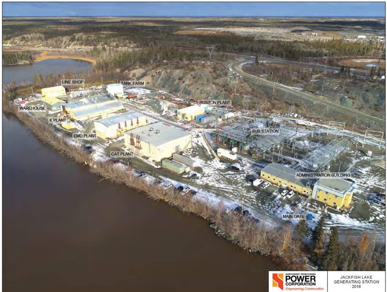
Figure 1-1: Jackfish Lake Generating Facility
