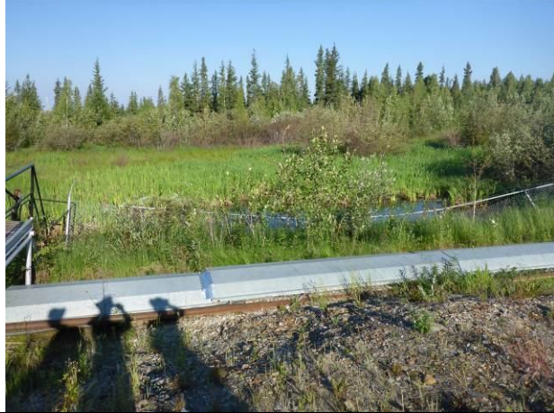
Photo #3: Overview of spill #16-153 location
