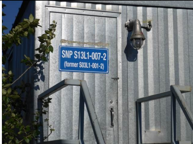
Photo #5: SNP signage located at the discharge of the backwash pond to the Mackenzie River
