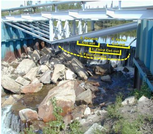
**Photo E: Bosworth Creek Lower Bridge Following Weir Removal**
