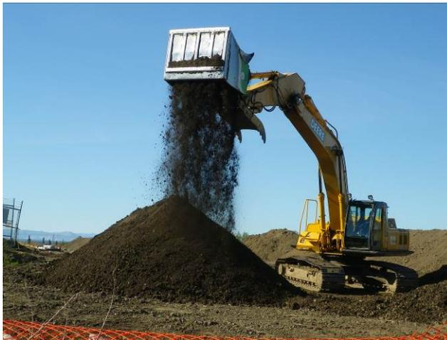
In 2012, the two smaller biocells were decommissioned and one larger biocell was reconstructed on the same site. The new biocell has a soil treatment capacity of approximately 5,000 m<sup>3</sup> (Imperial Oil 2013).
