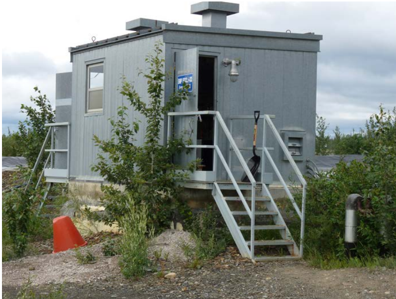
Photo C: Outlet Return Line Building and S03L1-02 Sampling Location
