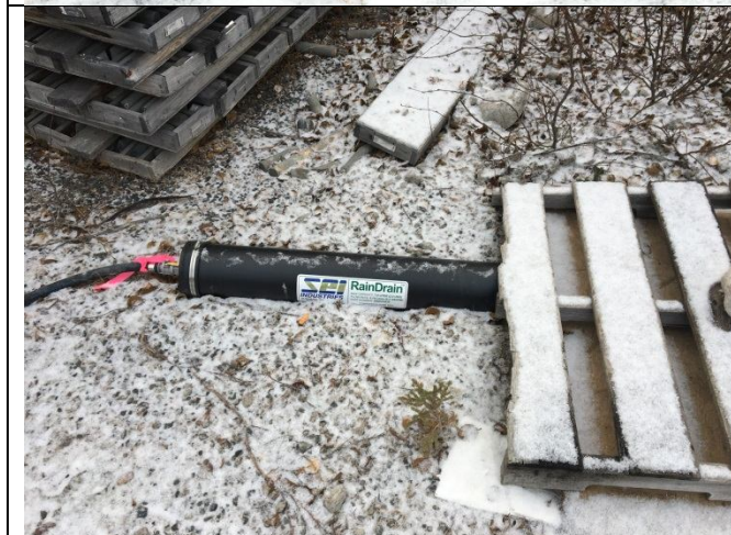
Photo #5: Water/Fuel separator. The RainDrain filter automatically removes rainfall and water collected inside a berm while also holding back hydrocarbons from the environment. Using gravity to filter the hydrocarbons out of rainwater, the RainDrain allows operators to safely drain overflow from their berms (berms need to remain empty to have the capacity to contain any spills).
