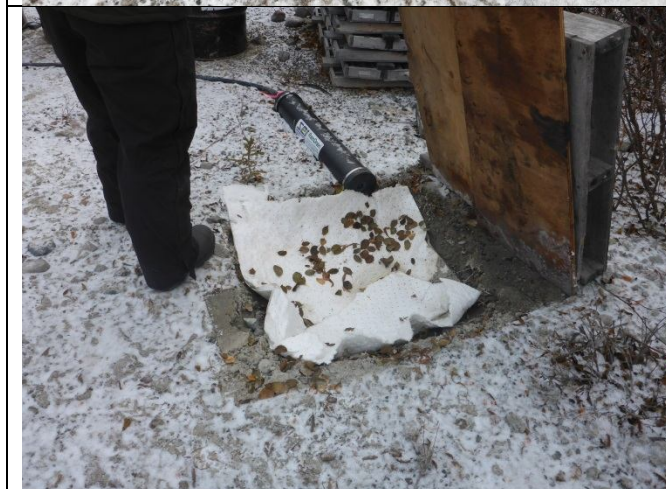
Photo #6: Soak away sump used to allow water to drain into the ground.
