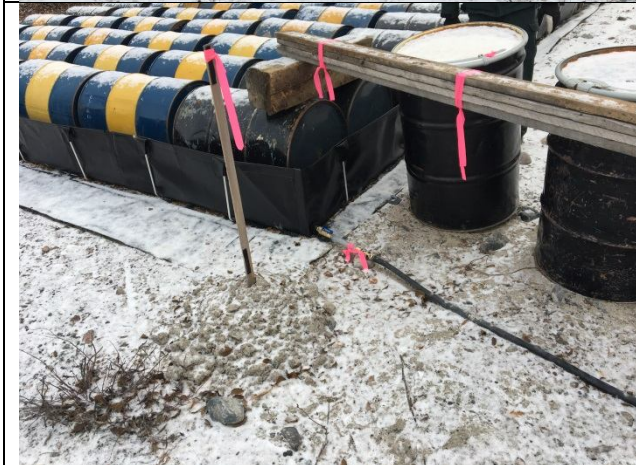
Photo #2: DEMCo Fuel Cash inside secondary containment.
