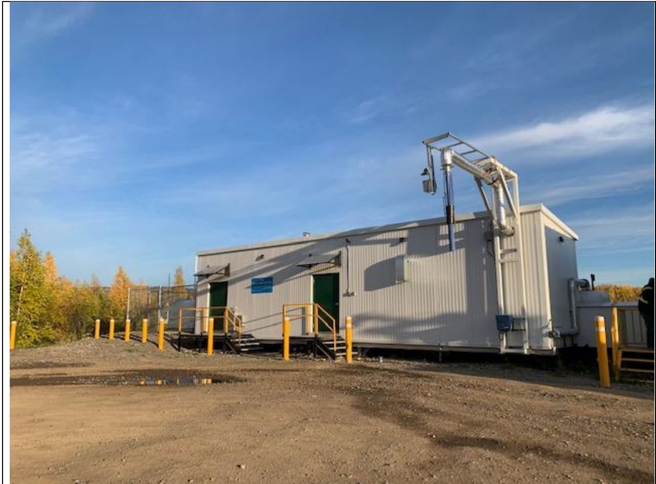
Figure 1: Water Intake Facility
