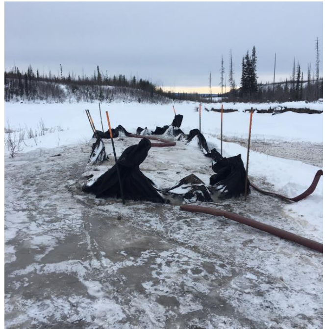
Figure 4 – Backfilled Dig Pit
