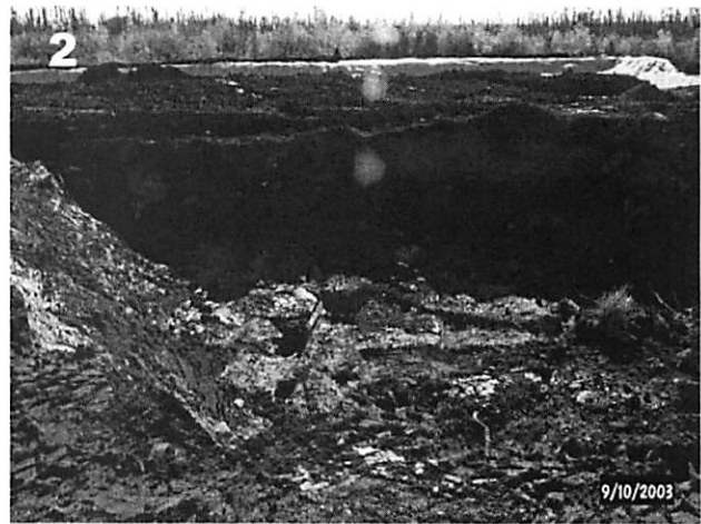
Excavation at FTA site
