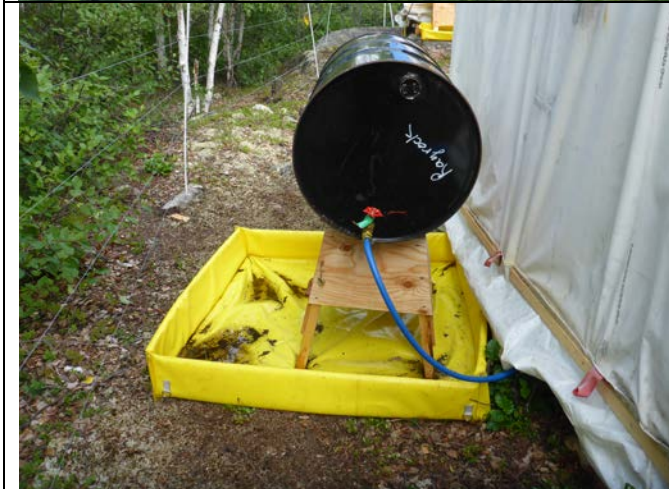
Photo #3: Heating fuel barrel connected to one of the camp tents
