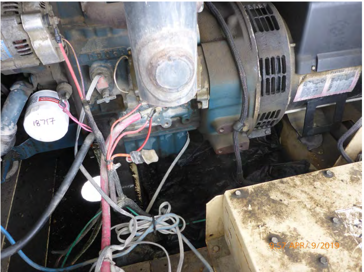
Photo 4 – Sable Laydown – This drip tray has spill pads that have become saturated with oil and will need to be addressed. Dominion has submitted a follow-up email to the Inspector indicating that this concern had been addressed shortly after the inspection.
