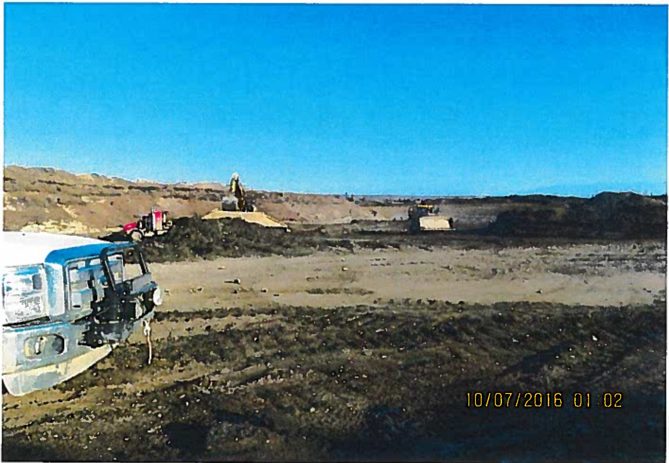
Loading trucks with gravel
