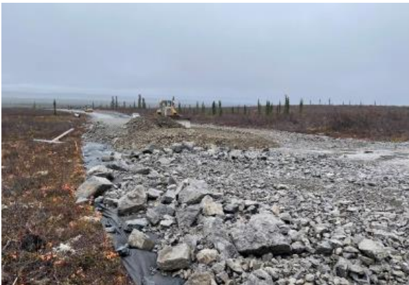
Spread & Compaction of Embankment Material
