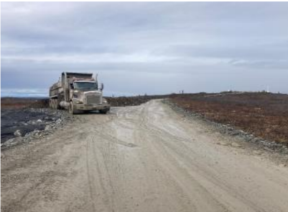
Dumping Embankment Material
